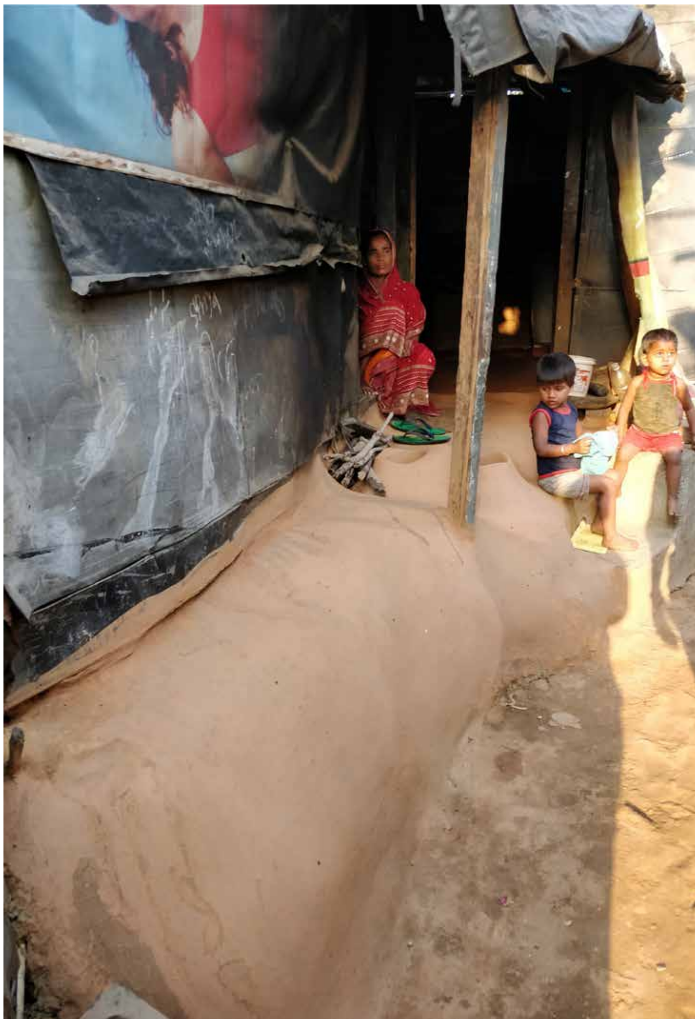
Floors made of mud plaster
