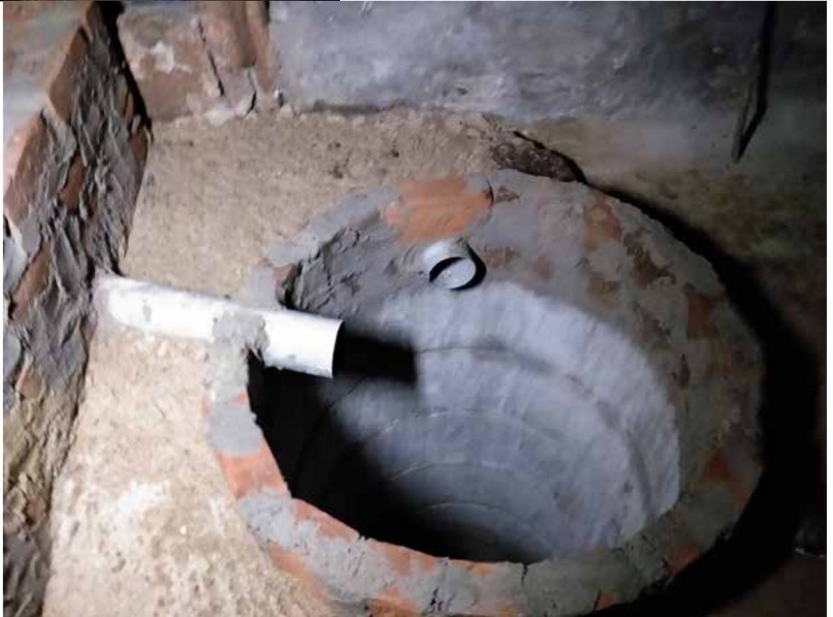
People are building toilets with a single septic tank made of concrete rings.
