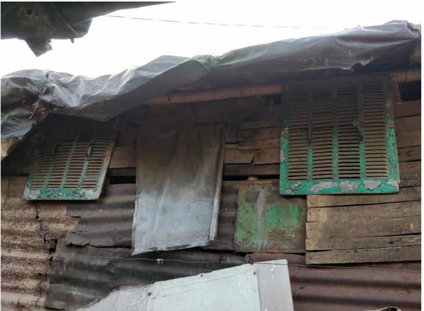
Air cooler covers are used for covering the outer partition of house, also provides ventilation in the house.
