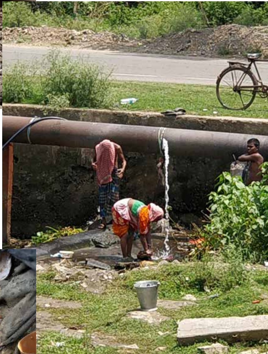
Stand post is constructed around leakage in the RMC water line
