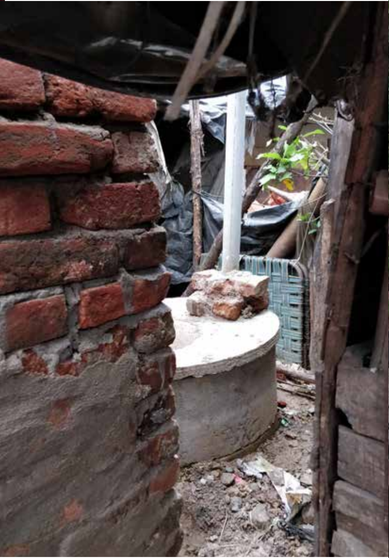
Toilet constructed in one of the house with concrete ring septic tank.
