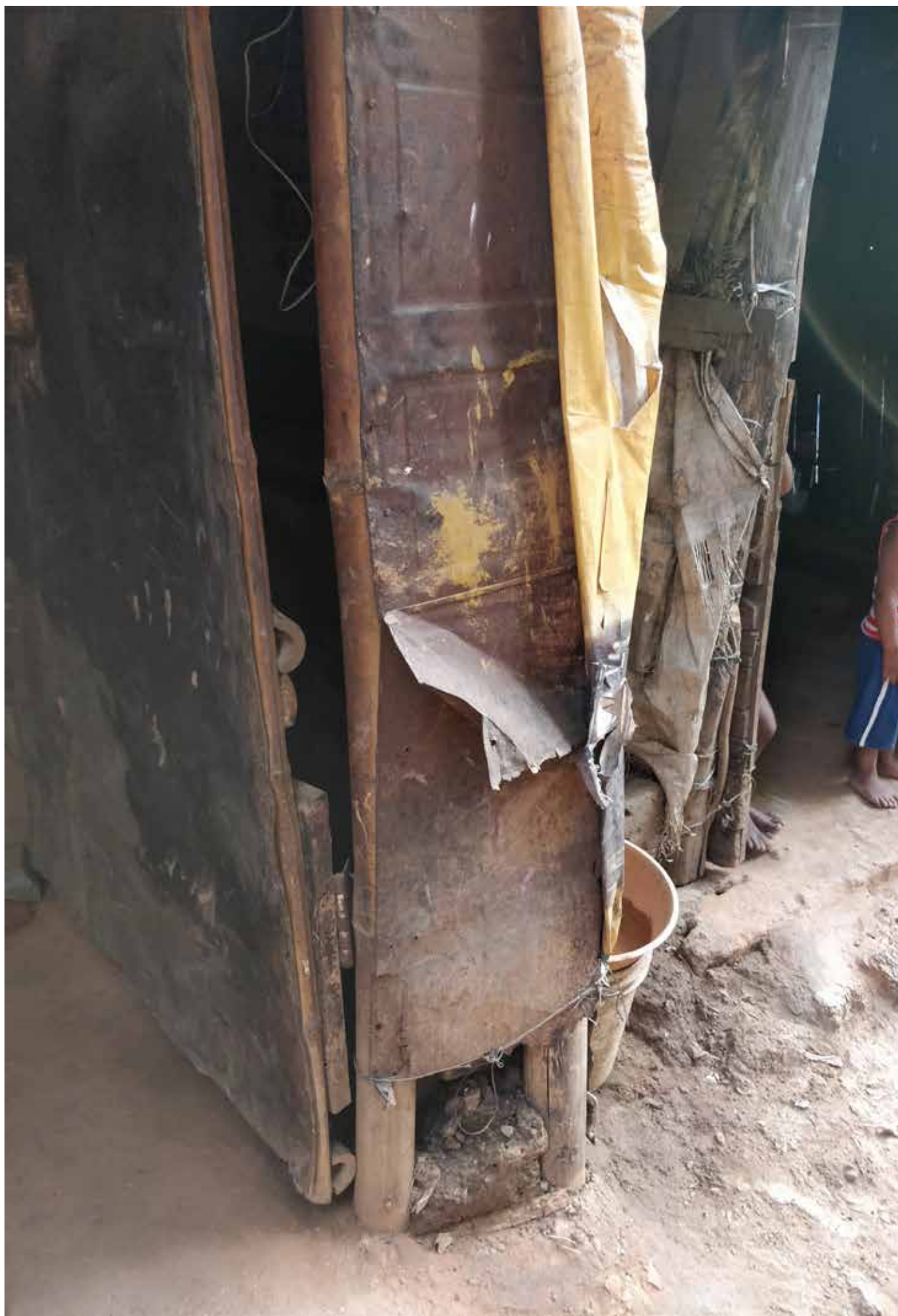
House wall partition detail - made of Bamboo framing and tin covering
