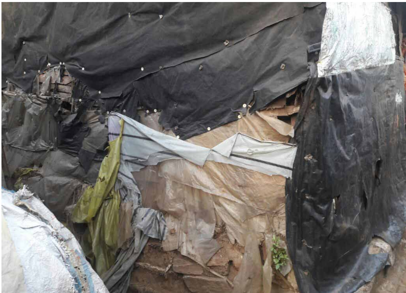
Exterior walls of the house is covered with tarpaulin sheet to avoise seepage of water during rains.
