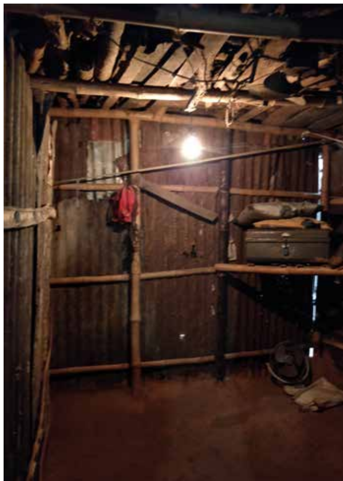
Partitions made of bamboo structure and tin covering
