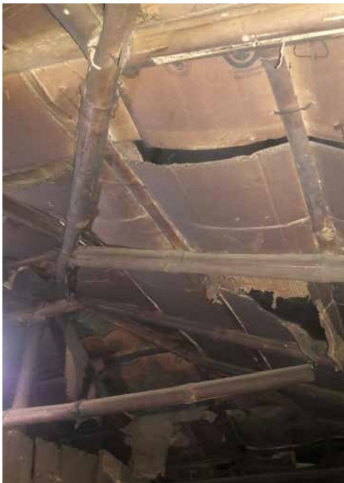
Roof made of bamboo structure and cardboard and tarpaulin sheet covering
