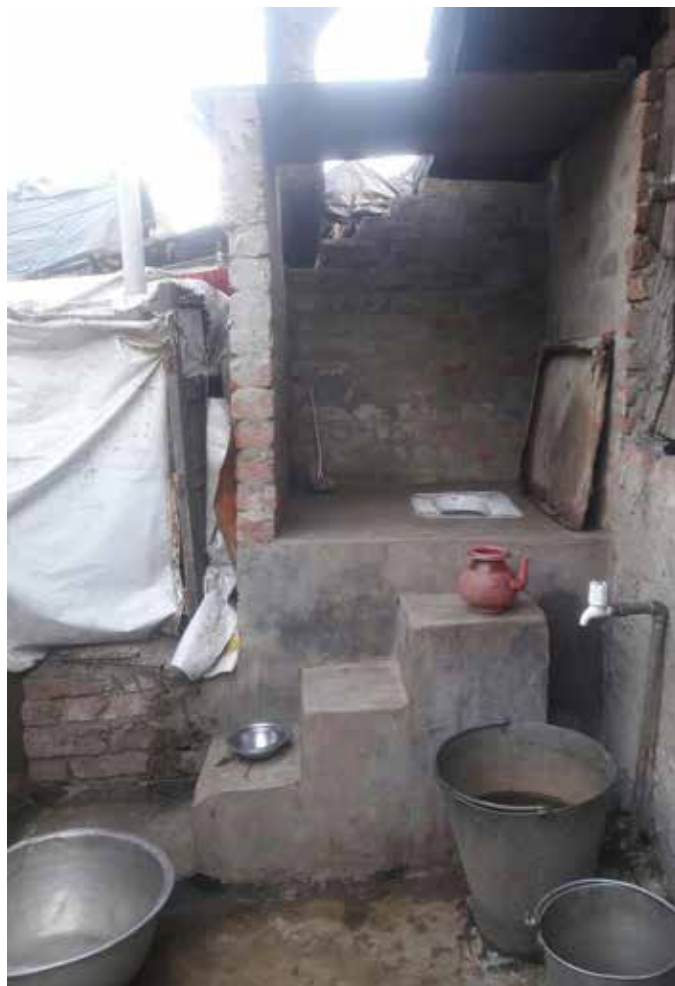
Toilet constructed at the back of the house with septic tank , temporary roof and without door
