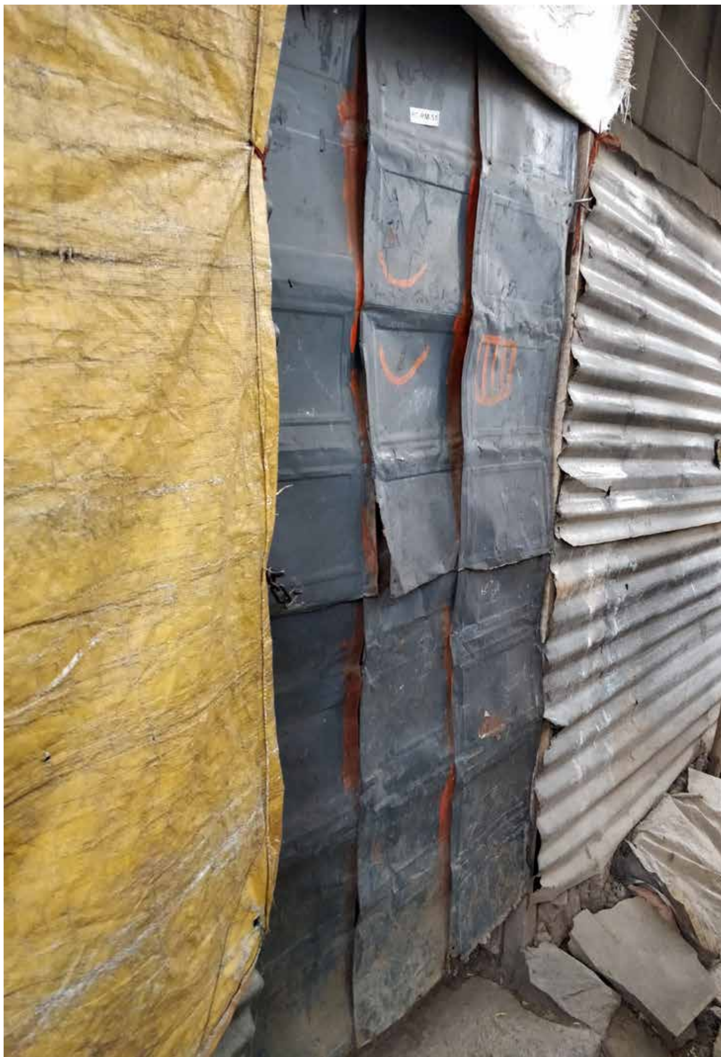
Doors made of Bamboo framing and waste tin cans
