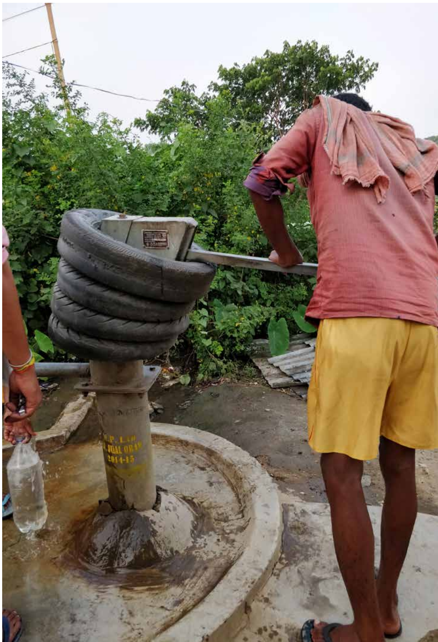
Tyres are used to avoid damage of handpump handle while withdrawing water from it.
